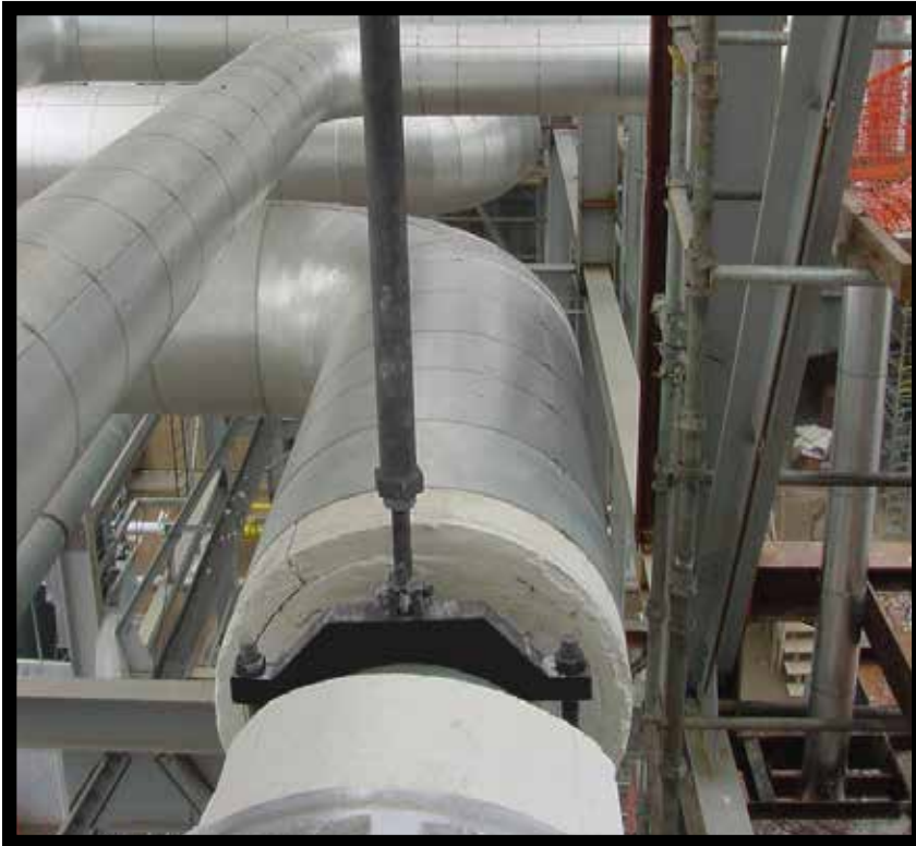
Rigid Strut with Fig RY3 stiff clamp
